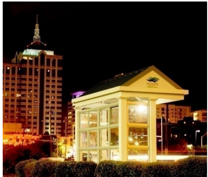
Figure 6-13: Updated Passenger Waiting Facility with Solar-Powered Lights
